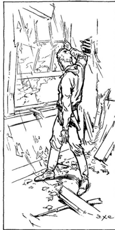
REGARDLESS OF FALLING TIMBERS AND CRASHING GLASS, THE ENGINEER CLUNG TO THE REMNANTS OF THE WINDOW
